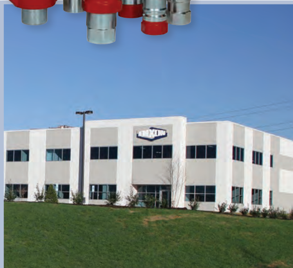
Dixon's 100,000 square foot facility in Dallas, NC supports manufacturing and warehouse functions.
